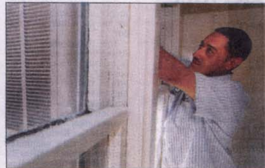
Ricardo Marin, a groundskeeper for the Housing Authority, works on an air-conditioning unit Thursday.
